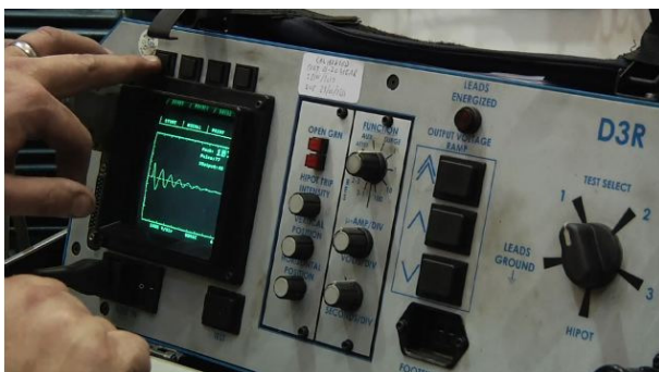
Baker surge comparison testing to ensure winding integrity
